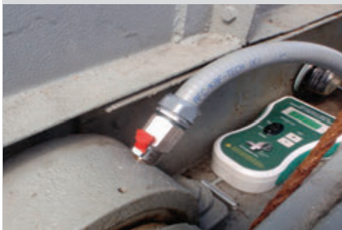
ADB Sensor Installed on Conveyor Bearing
